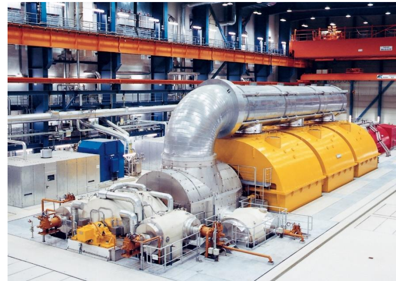
Multi-stage steam turbine + generator
