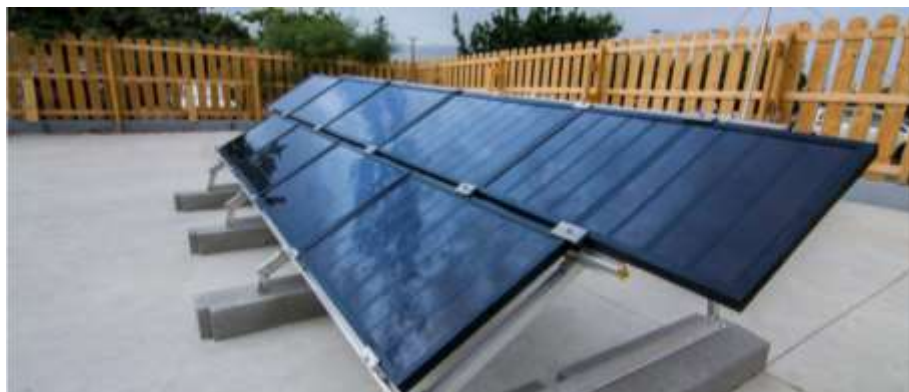
Figure 1: A photograph of the solar farm
