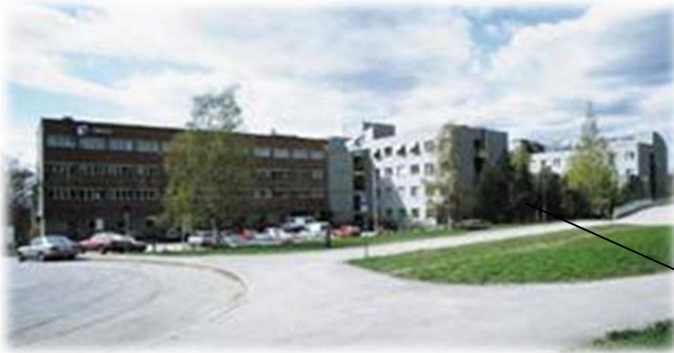
Labs and offices at Sintef, Oslo, Norway
