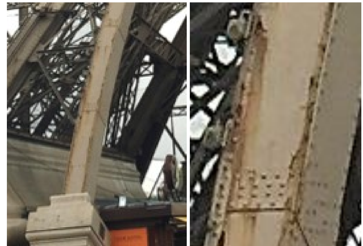
Alarming corrosion in Eiffel Tower, Paris, France
