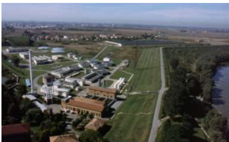
Figure 1: Pontelagoscuro Plant: near Ferrara, it treats Po river water on which there will be applied the innovative technology on emerging pollutants using graphene oxide
